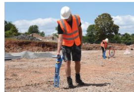
Safe underground infrastructure
