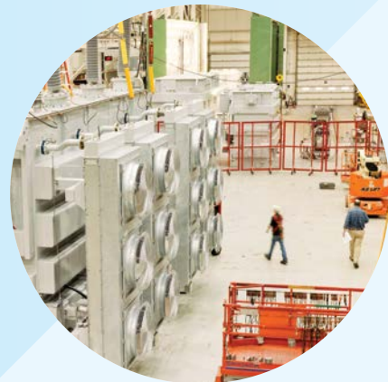
SPX Transformer Solutions— Waukesha Facility
