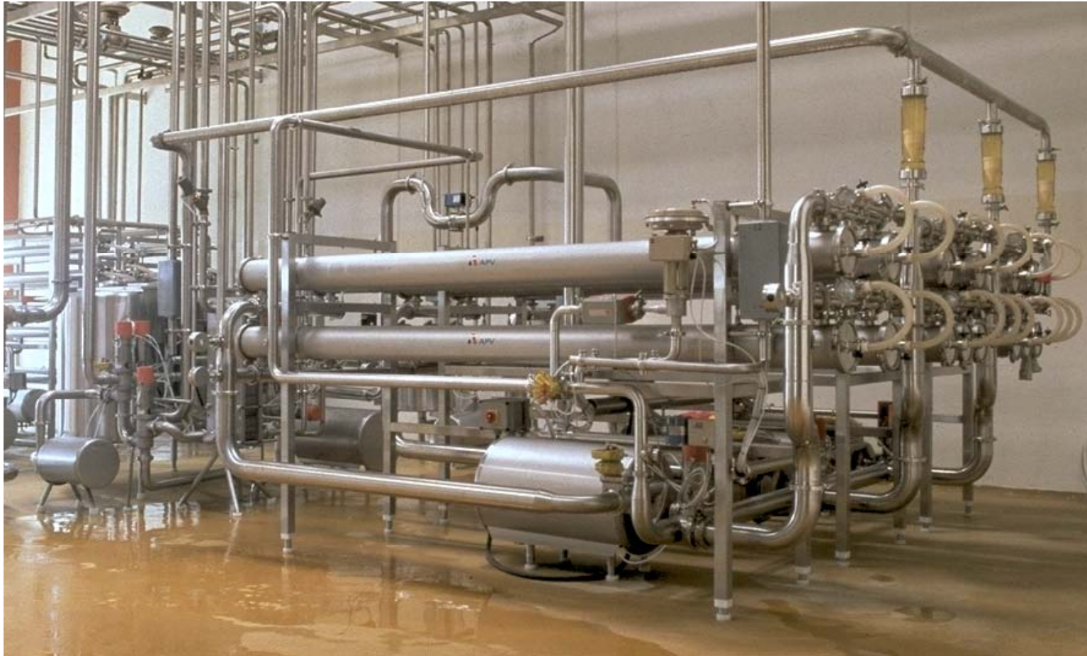
APV's Ultrafiltration System Used for the Treatment of Raw Milk At Arla Foods Cheese Production Facility in Sweden
