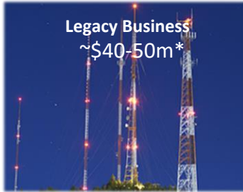
Flash Technology Terrestrial Obstruction Lighting
