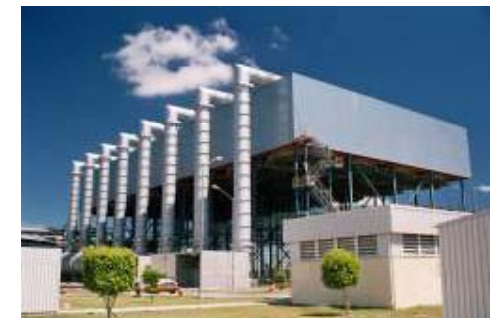
Dry Cooling System
