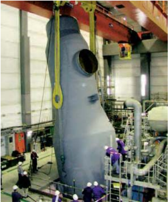
Moisture Separator Reheater for Nuclear Power Plants
