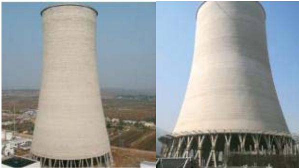
Indirect Dry Cooling Tower on Coal-Fired Power Plants in China
