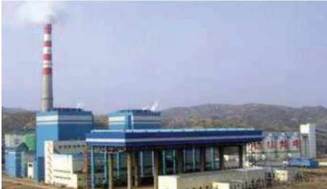
Air Cooled Condenser on a Coal-Fired Power Plant in China
