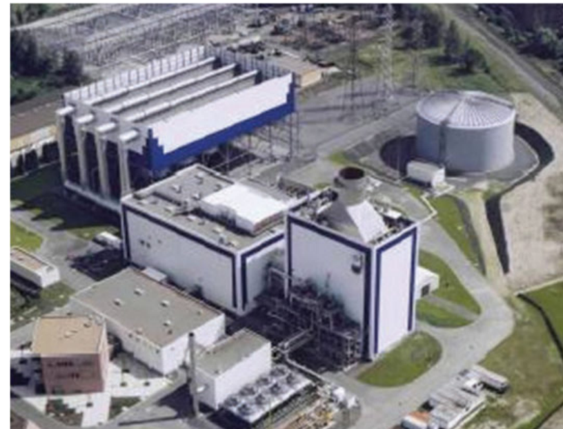
Natural Gas Power Plant in Europe
