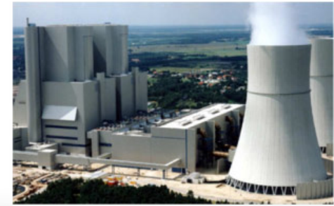
Coal Fired Power Plant in Europe
