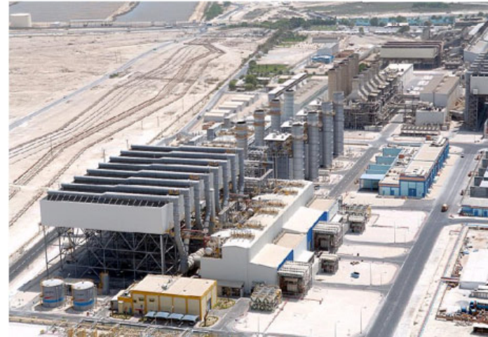
Natural Gas Power Plant in the Middle East
