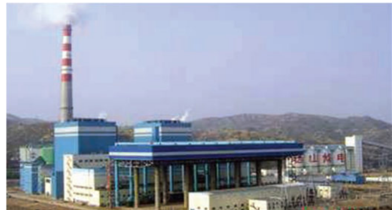
Coal-Fired Power Plant in China
