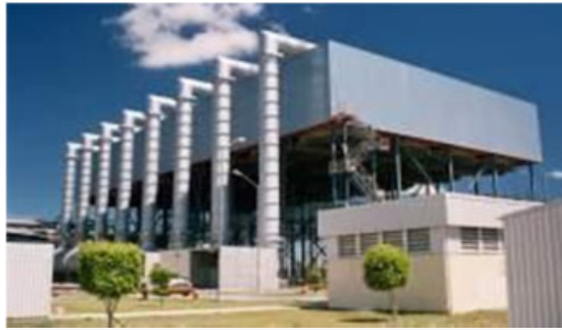
Natural Gas Power Plant in Mexico
