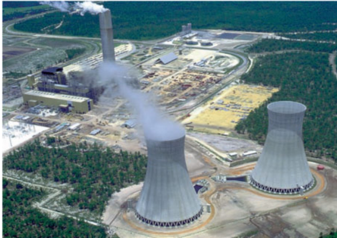
Coal-Fired Power Plant in the United States
