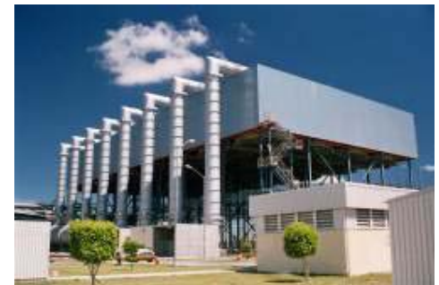
Dry Cooling System
