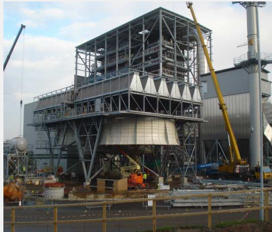
Dry Cooling (ModuleAir)
